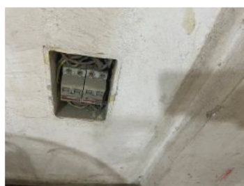
No insulation cover installed (2).JPG
