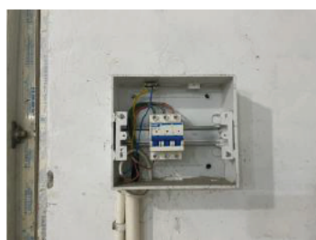
No insulation cover installed (3).JPG
